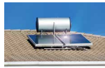
Installation on a sloping roof
