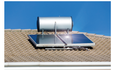
Installation on a sloping roof
