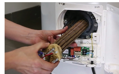
STEATITE no direct contact with the water -> element in a sheath
